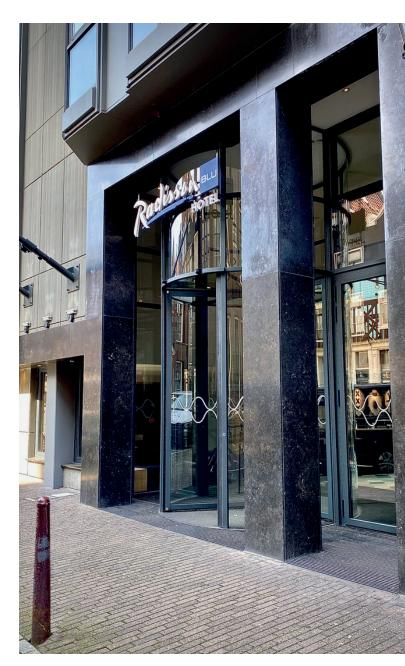
With this revolving door, security sensors have been placed on the corner parts of the door wings that look past the door wings. If the rotating part catches up with the passer-by while turning and the passer-by enters the security field, the rotating part will stop. If the passer-by moves out of the security field, the rotating part will start up again.
